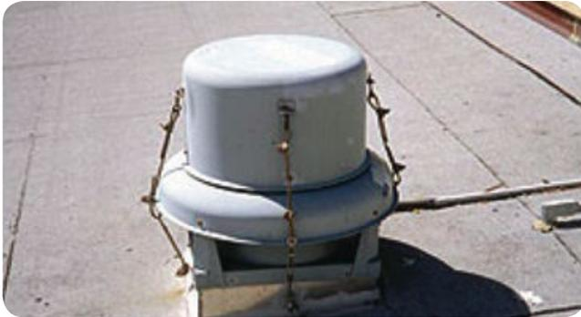
Use of securement straps – several fasteners should be used.
